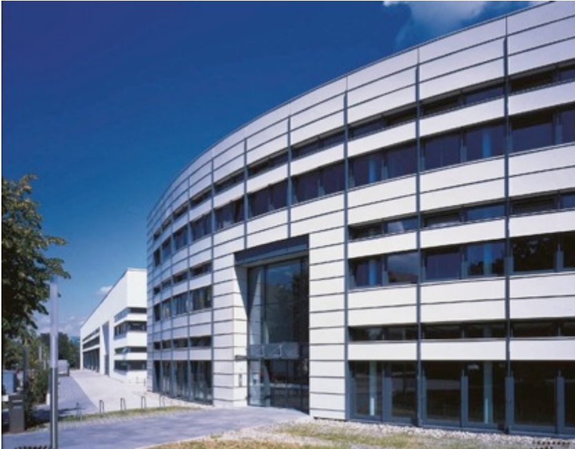
Headquarter of Fraunhofer ISE, Freiburg, Germany
