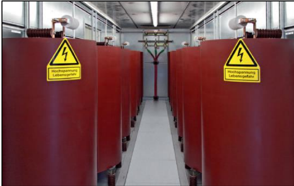
Fig 1: Inside a 6 MVA LVRT and grid decoupling unit
