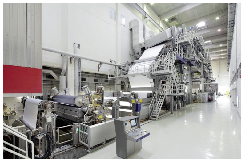
PICTURE 1 Coating machine with condition monitoring at Mitsubishi, Bielefeld
