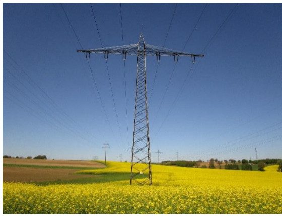
The control and maintenance of overhead lines will be supported by AI in the future
