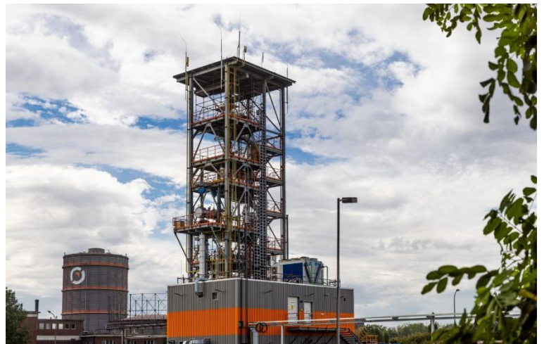
μDRAL plant — first direct reduction plant flexibly operated with hydrogen and natural gas in an integrated mill.
